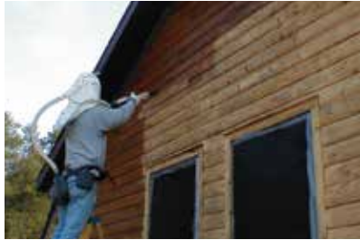
Blast Cleaning & Restoration
